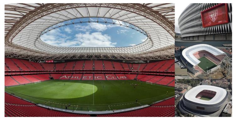
The stadium is located in Calle Felipe Serrate and will seat some 53,500 spectators. The plan shape is practically oval measuring  $220 \times 174$ m. The stadium is to be constructed in two phases to allow the use of the current stadium until the end of the phase of the new one. It is divided into twelve sections connected by expansion joints.
